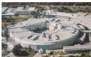
Elettra, Italy (2009) 2 GeV
